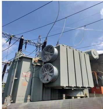
**Gambar 4 Transformator IBT Daya 100 MVA**
