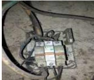
Gambar 2. MCB (*Miniature Circuit Breaker*)
