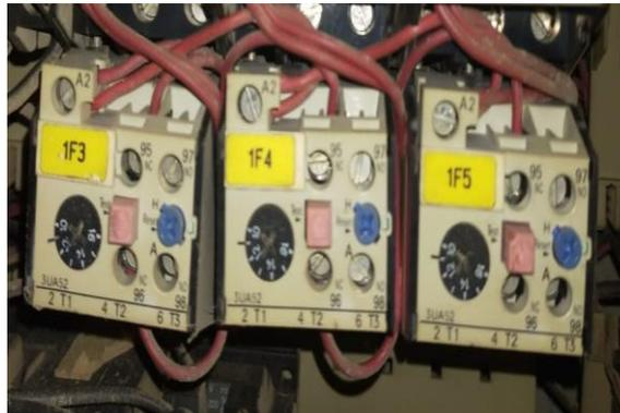
Gambar 5. *Thermal Over Load (TOR)*
