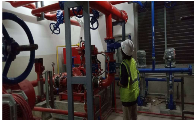
Gambar 18b. Pompa Electrical Hydrant Pump (Sumber PT. JAGA CITRA INTI) Diesel Hydrant Pump
