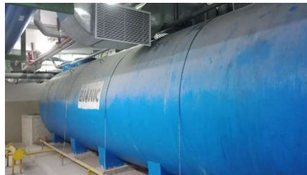
Gambar 14. GWT ( Ground Water Tank ) Bionic (Sumber Pribadi)
