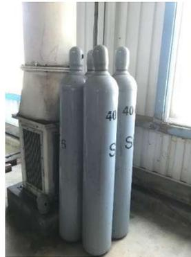
**Gambar 2.** Gas SF<sub>6</sub> (Sulfur Hexafluoride)
